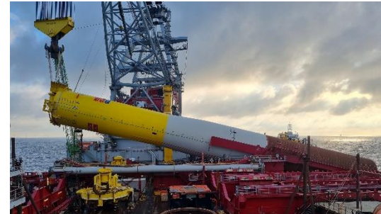
LiftLOK™ Lift and installation
